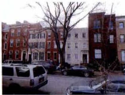
6 OPP. SIDE OF STREET - EXISTING A6 SCALE: NO SCALE
