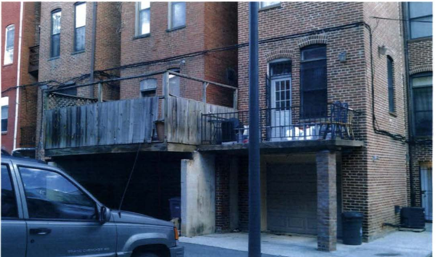
Back of neighboring houses (lots 94 and 95). These decks/porches are not original to the main structure and were constructed at a later date. Aside from these decks, the subject house and its neighbors were constructed at the same time, have identical lot sizes, the same configuration, and lot occupancy.
