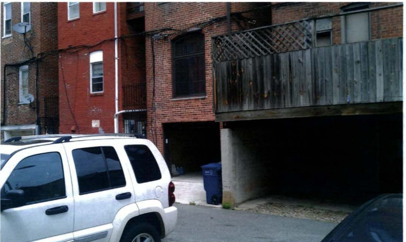
Back of house (lot 93) at alley. View looking Northeast. Imposing deck at right (lot 94).
