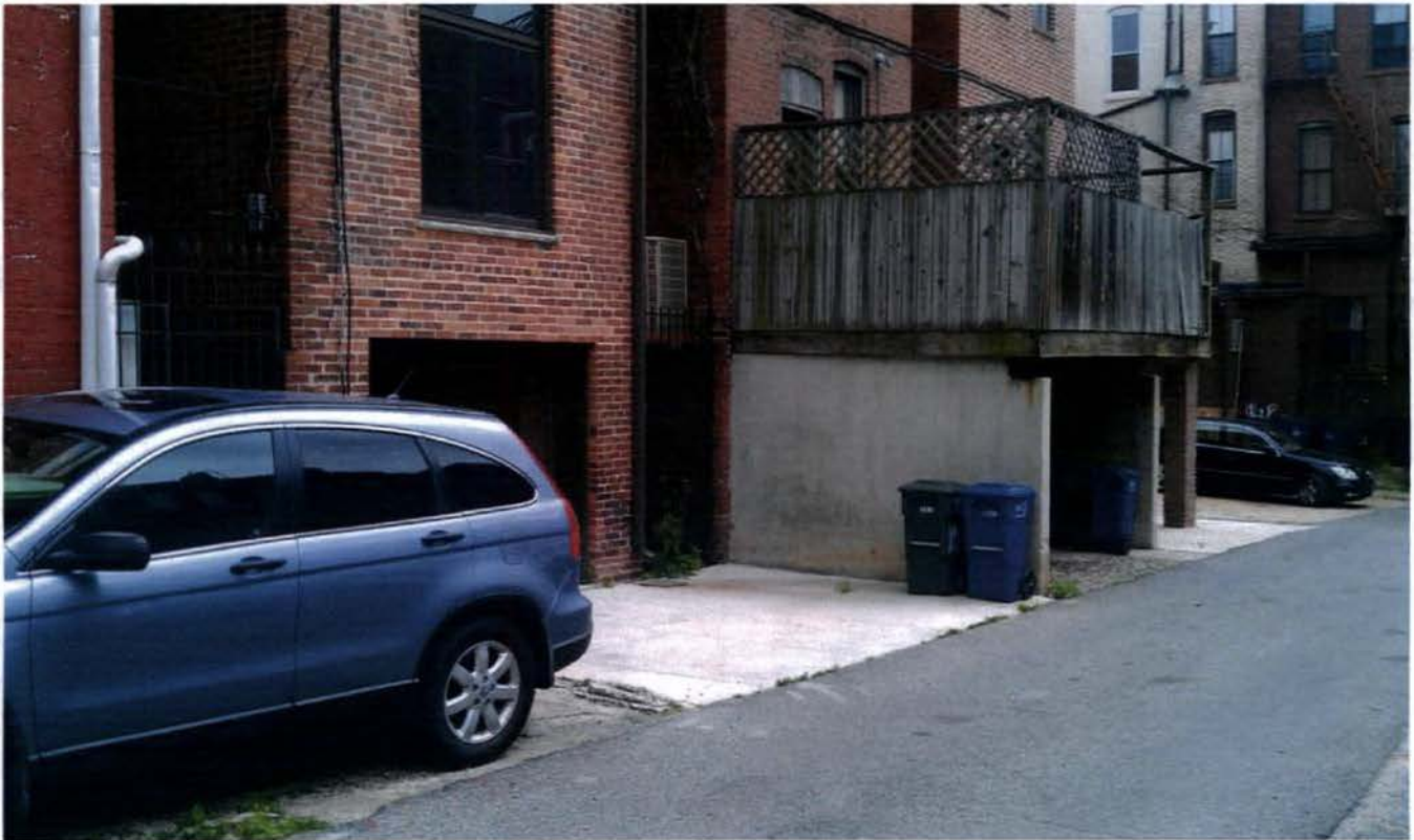
Back of house (lot 93) at alley. View looking Southeast. Neighbor's deck structure beyond (lot 94).
