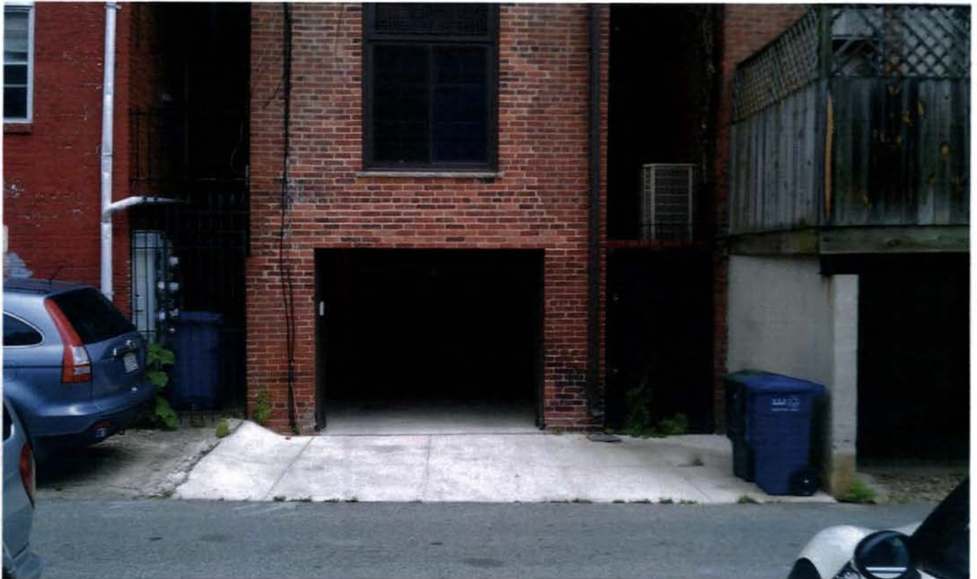
Back of house (lot 93) at alley. View looking East. Neighbor's deck structure at right (lot 94).
