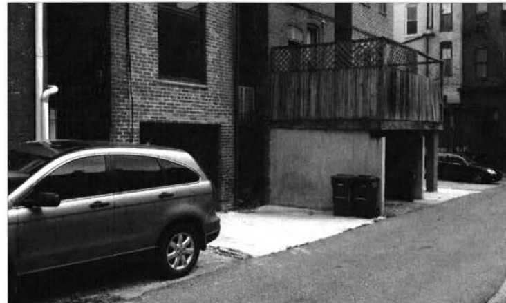
EXISTING REAR YARD CONDITION AT ALLEY
