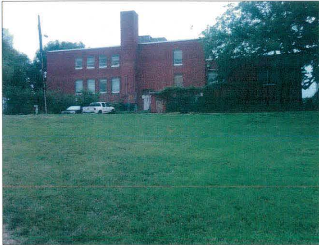
View of site looking north across Langdon Park
