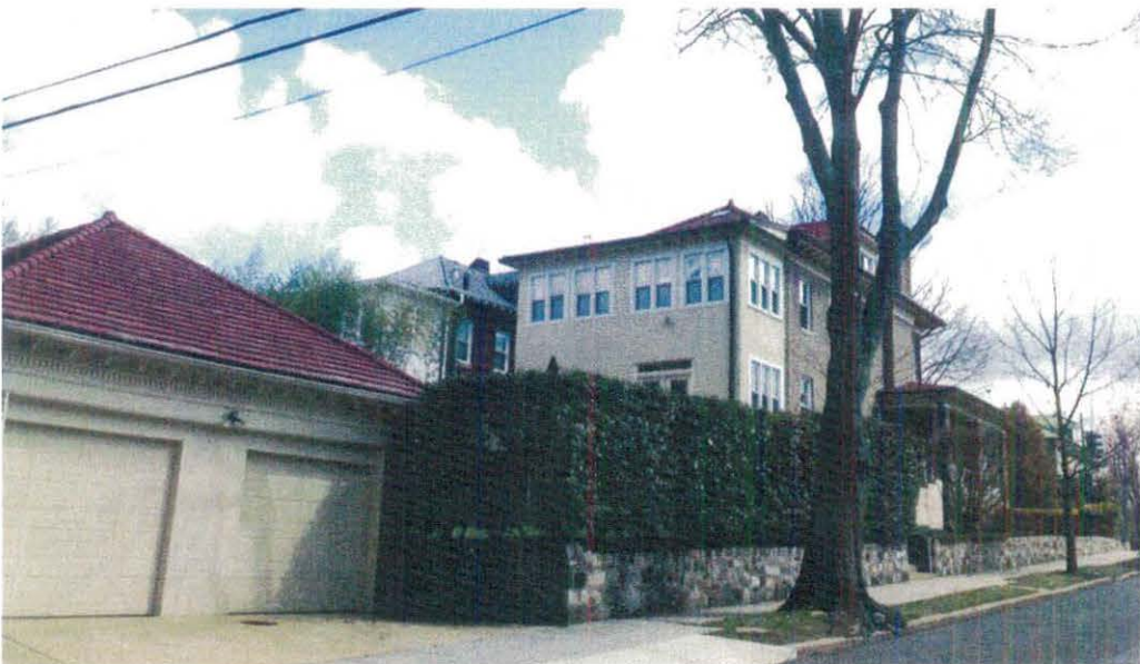
Rear View From Montague Street
