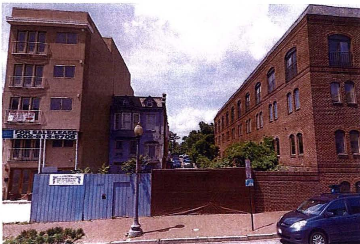
View from Wisconsin Avenue, NW- the Subject Property is behind the brown wooden wall
