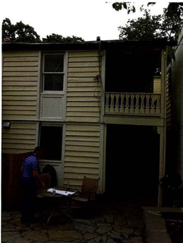
VIEW TO TWO STORY BRICK HOME - EAST
