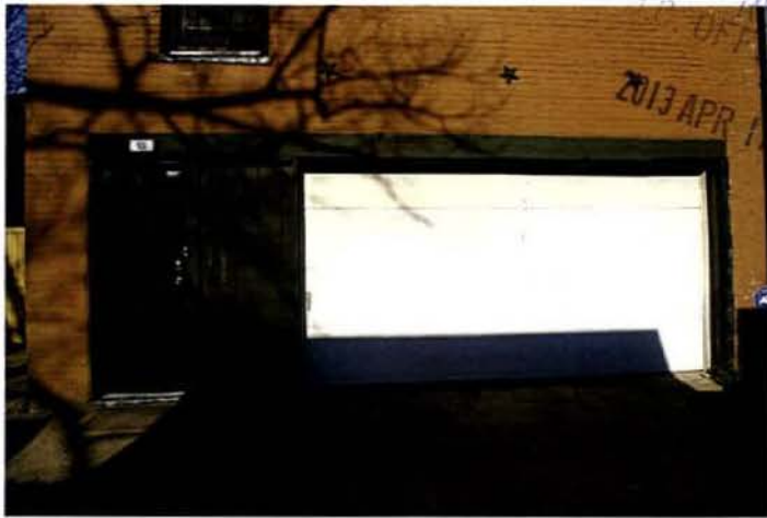
VIEW OF GARAGE BLDG. IN THE AREA
