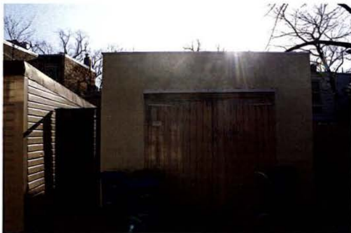
STORAGE STRUCTURE - EAST
