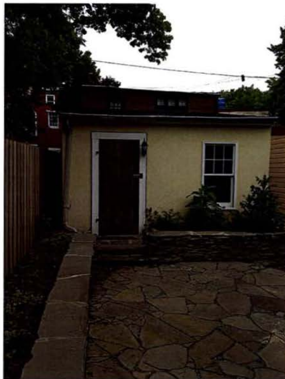
STORAGE STRUCTURE - WEST
