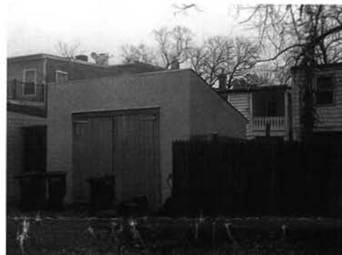
4 EXISTING PHOTO - STORAGE STRUCTURE EAST
