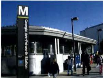
GEORGIA AVE / PETWORTH METRO STATION
