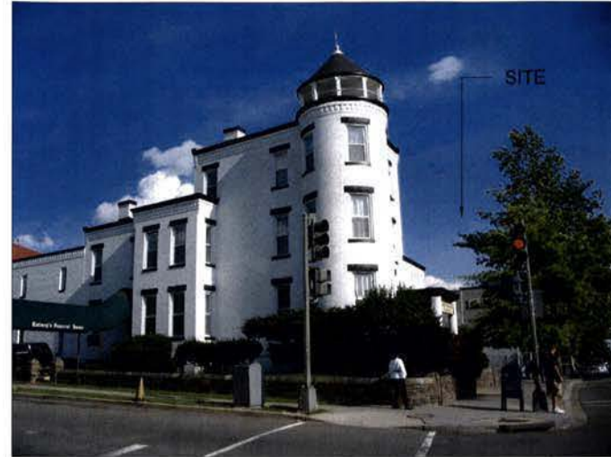
② RANDOLPH STREET (LOOKING SOUTH)
