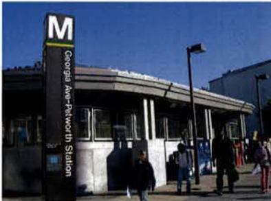
GEORGIA AVE / PETWORTH METRO STATION
