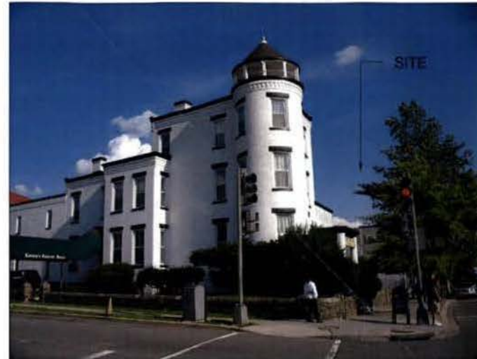
② RANDOLPH STREET (LOOKING SOUTH)
