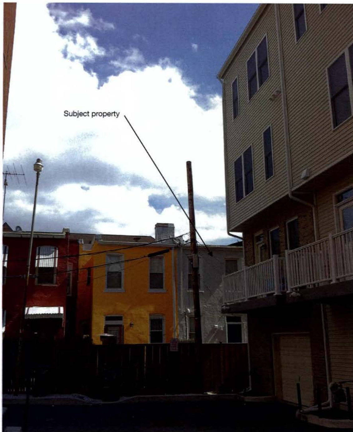
Figure 3. Rear view of subject property from alley.
