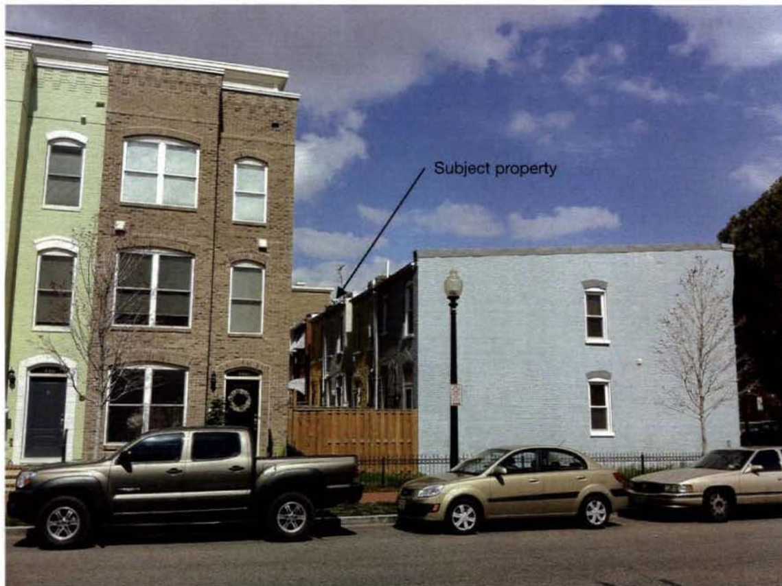
Figure 5. Side view of subject property and block from south.
