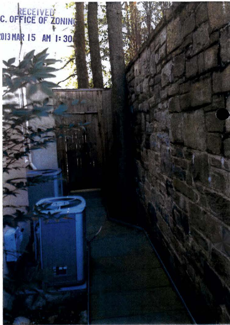
SY WEST FACING FRONT HOUSE
