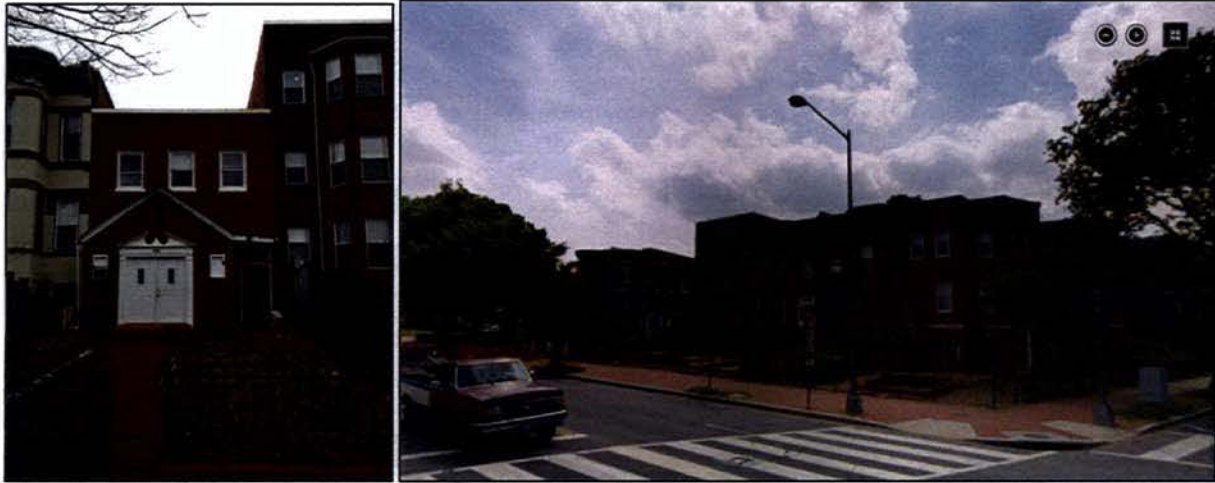
FRONT OF PROPERTY FROM NEW JERSEY AVENUE, NW
