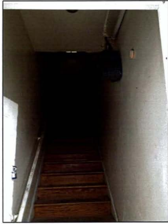
STAIRWELL LEADING TO 2 ND FLOOR APT.
