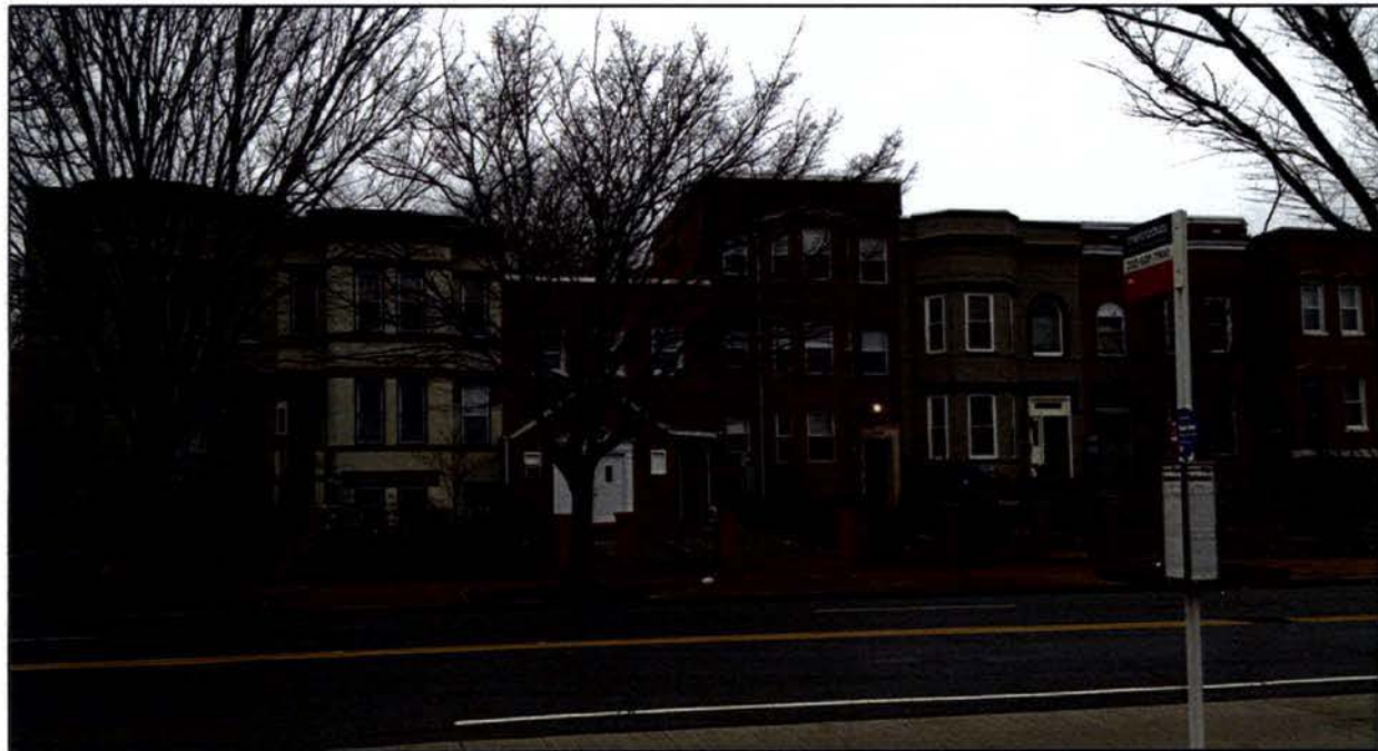
FRONT OF PROPERTY FROM NEW JERSEY AVENUE, NW
