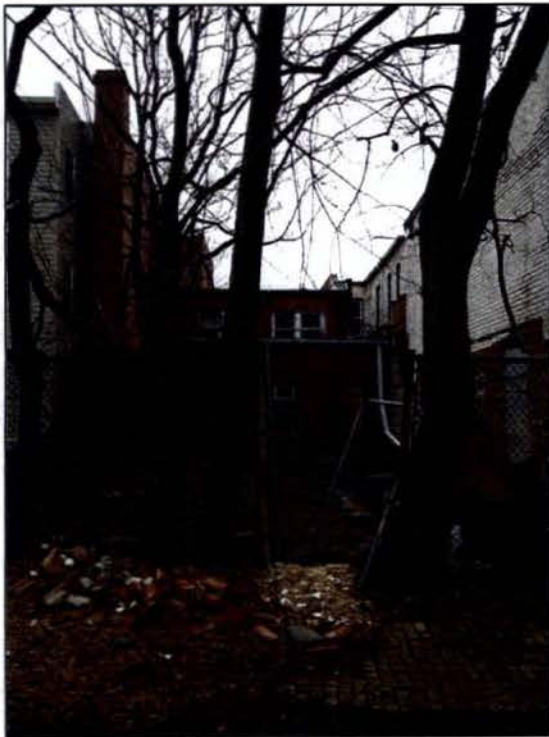
REAR OF STRUCTURE
