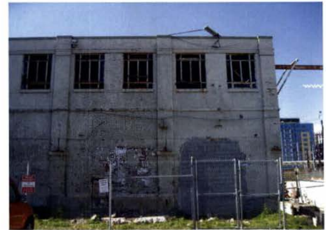
EAST FACADE SECOND STORY ADDED IN 1936
