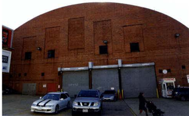
NORTH FACADE FROM M STREET NE
