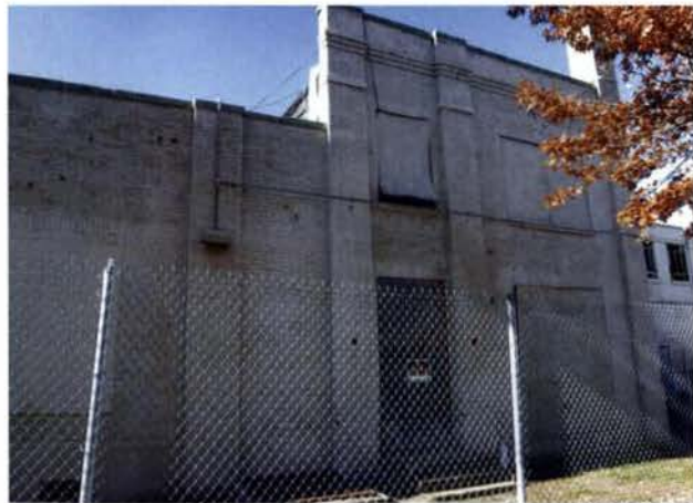
EAST FACADE 2ND STORY OFFICE ADDED IN 1934
