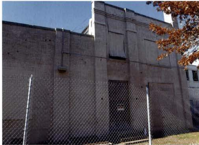
EAST FACADE 2ND STORY OFFICE ADDED IN 1934
