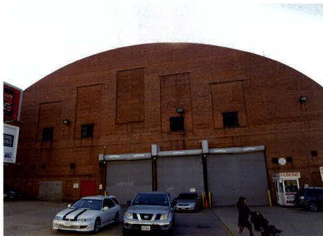
NORTH FACADE FROM M STREET NE
