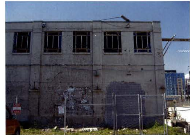
EAST FACADE SECOND STORY ADDED IN 1936
