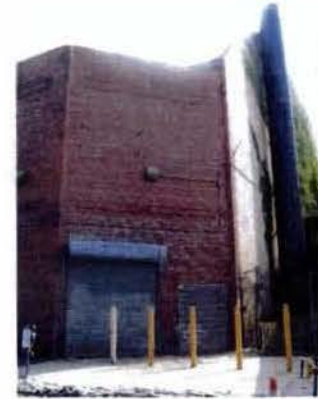
6 EXISTING LOADING DOCK
