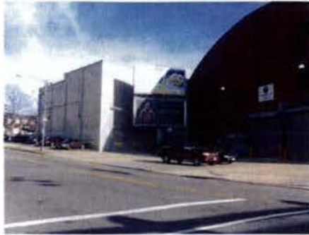
1 ICE HOUSE AND ADJACENT ARENA
