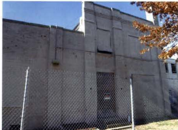
EAST FACADE 2ND STORY OFFICE ADDED IN 1934
