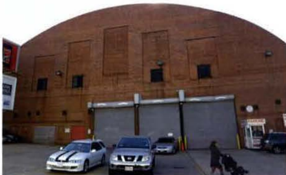
NORTH FACADE FROM M STREET NE
