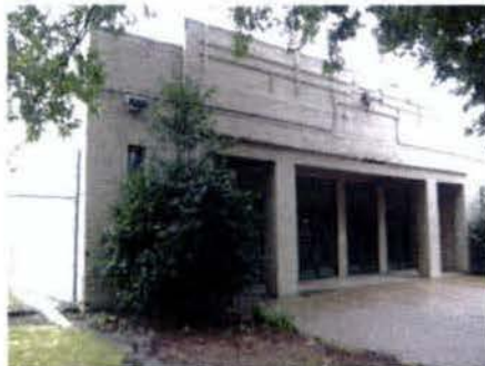
3 ICE HOUSE MAIN ENTRANCE
