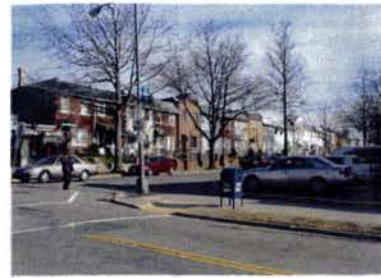
3 M STREET LOOKING SOUTHEAST
