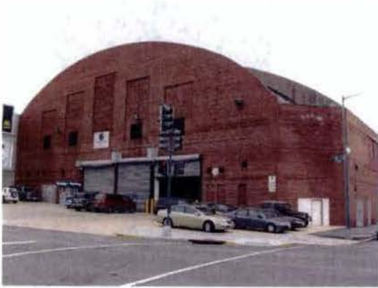
1 ARENA MAIN ENTRANCE
