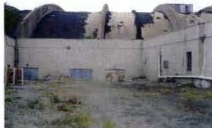
5 VIEW OF ARENA ROOF FROM 3RD STREET
