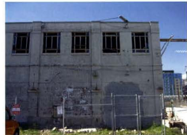
EAST FACADE SECOND STORY ADDED IN 1936
