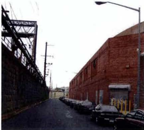
2 DELAWARE AVENUE LOOKING NORTH
