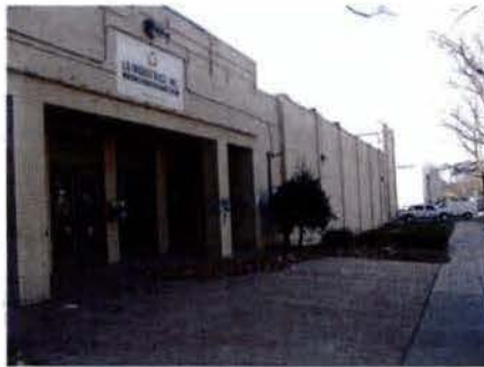
2 ICE HOUSE MAIN ENTRANCE
