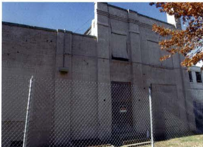
EAST FACADE 2ND STORY OFFICE ADDED IN 1934
