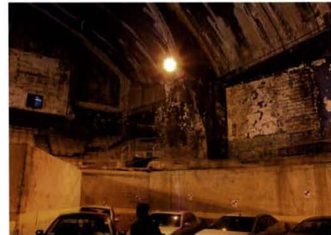
NORTH EAST CORNER ADJACENT TO ICE HOUSE
