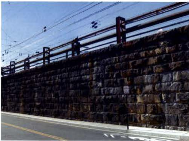
ELEVATED TRACKS IMMEDIATELY WEST OF SITE
