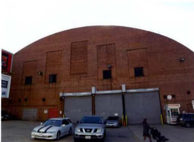
NORTH FACADE FROM M STREET NE
