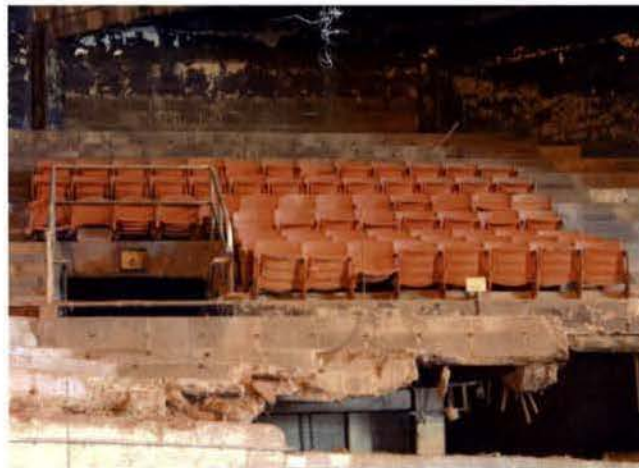
EXISTING STANDS SOUTH WEST CORNER
