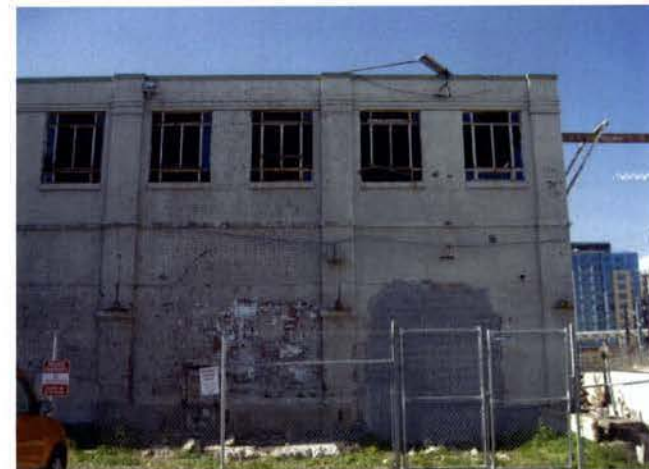
EAST FACADE SECOND STORY ADDED IN 1936
