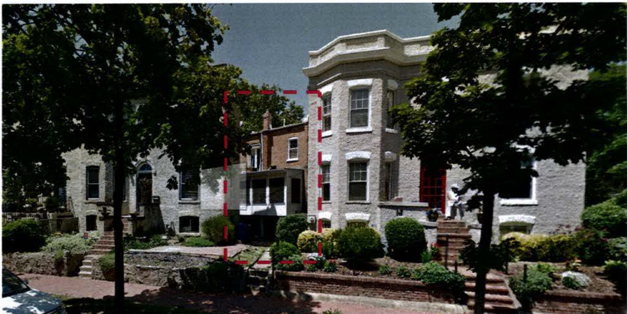
View of enclosed porch from Independence Avenue.
