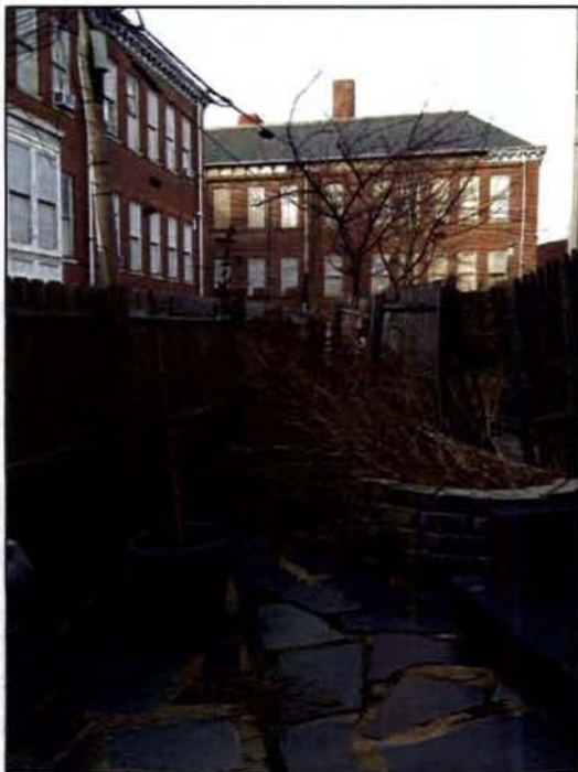
REAR OF STRUCTURE FACING NORTH INTO REAR YARD
