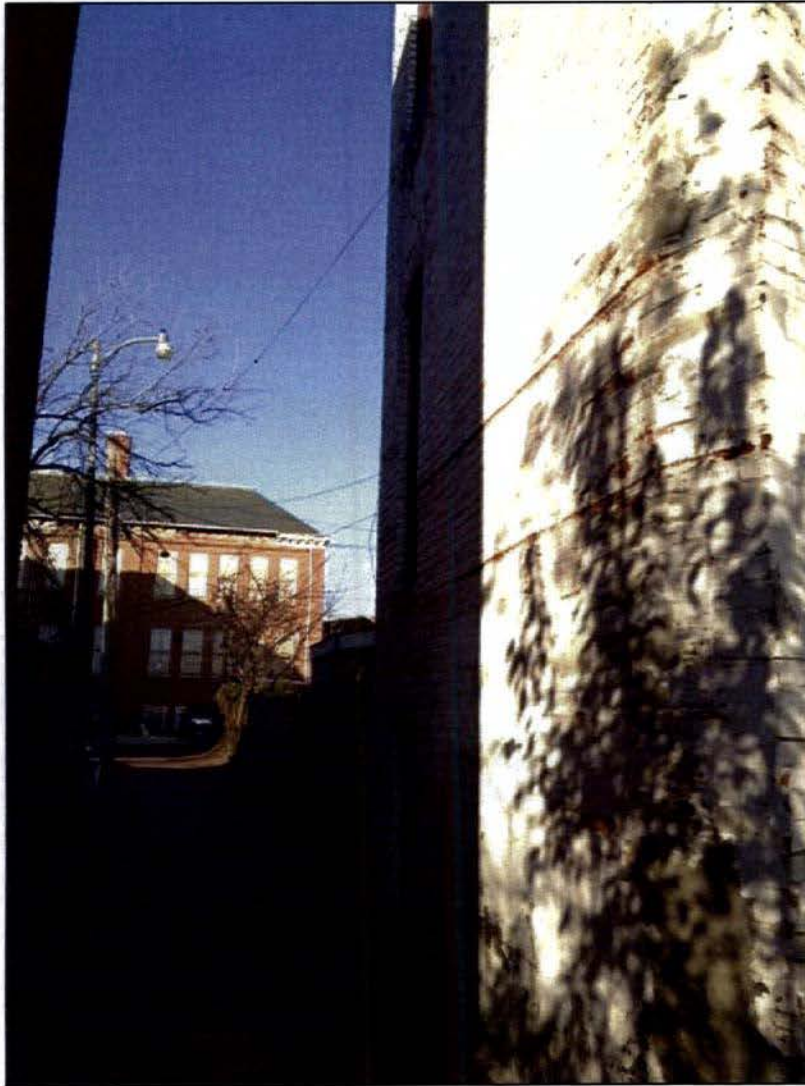
WEST SIDE OF STRUCTURE FROM ALLEY FACING NORTHEAST
