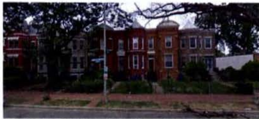
2. ADJACENT PROPERTIES ALONG MARYLAND AVE NE
