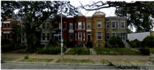
2. ADJACENT PROPERTIES ALONG MARYLAND AVE NE
