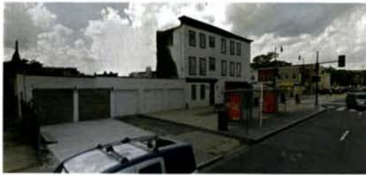
1. ADJACENT PROPERTY ALONG 14TH ST NE
