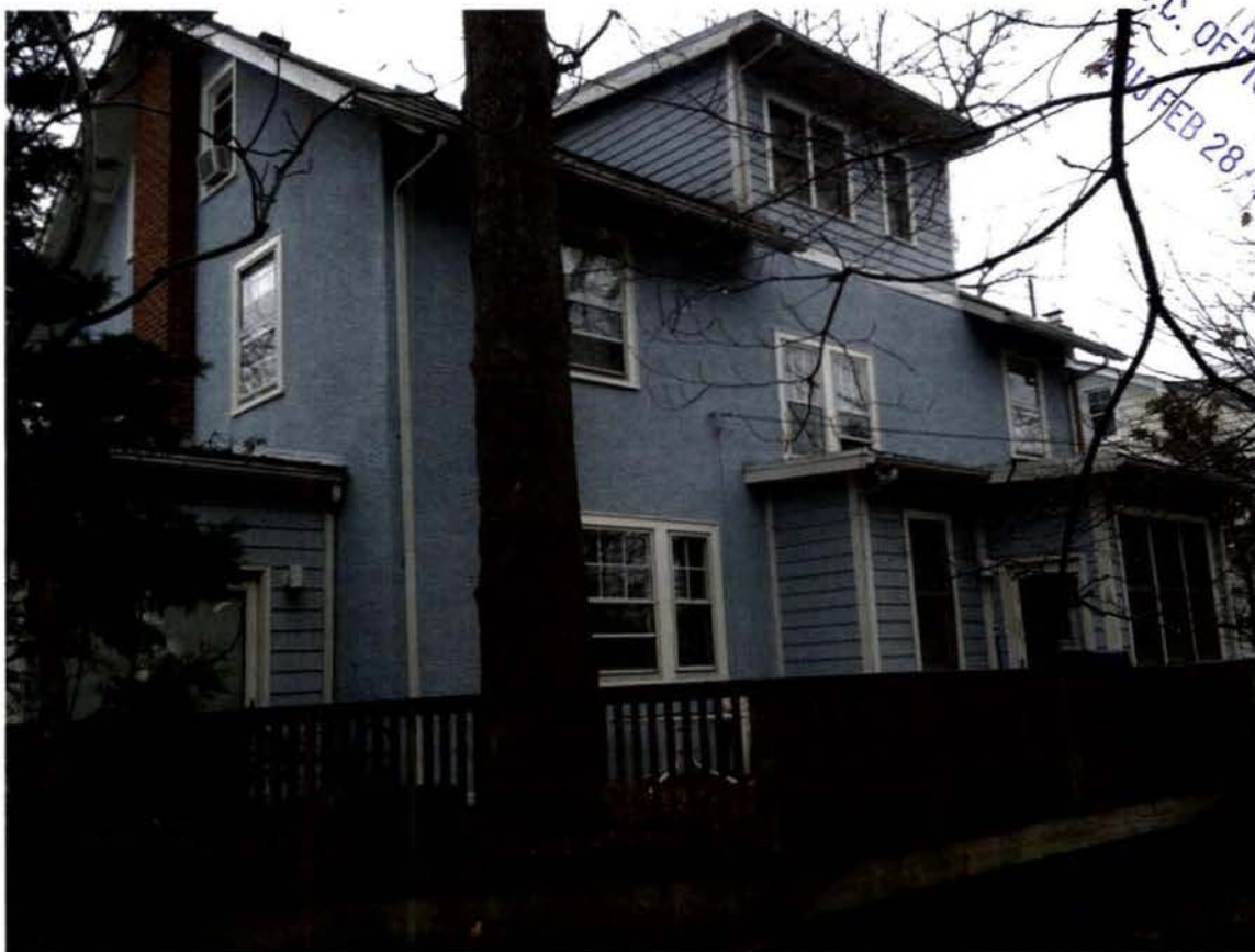
Existing View from Rear (North East)
