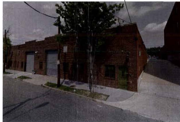
2. FRONT VIEW FROM SHANNON PLACE ST. LOOKING TOWARDS ALLEY
