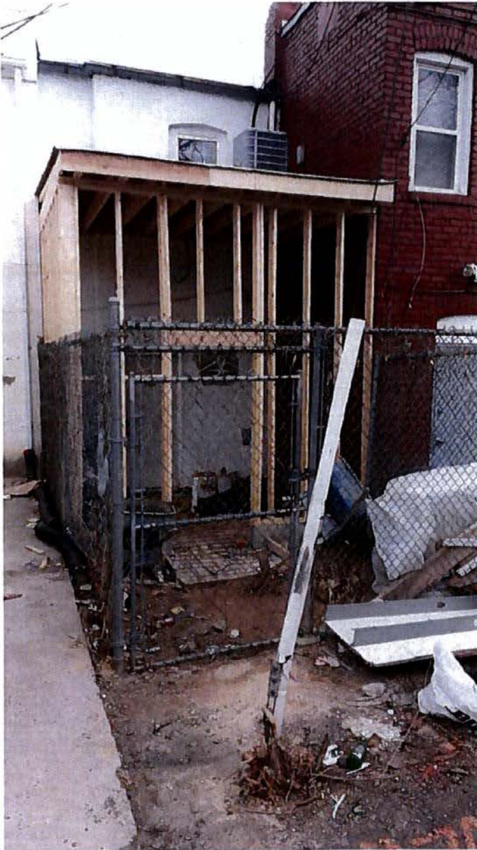
The rear of the Property
