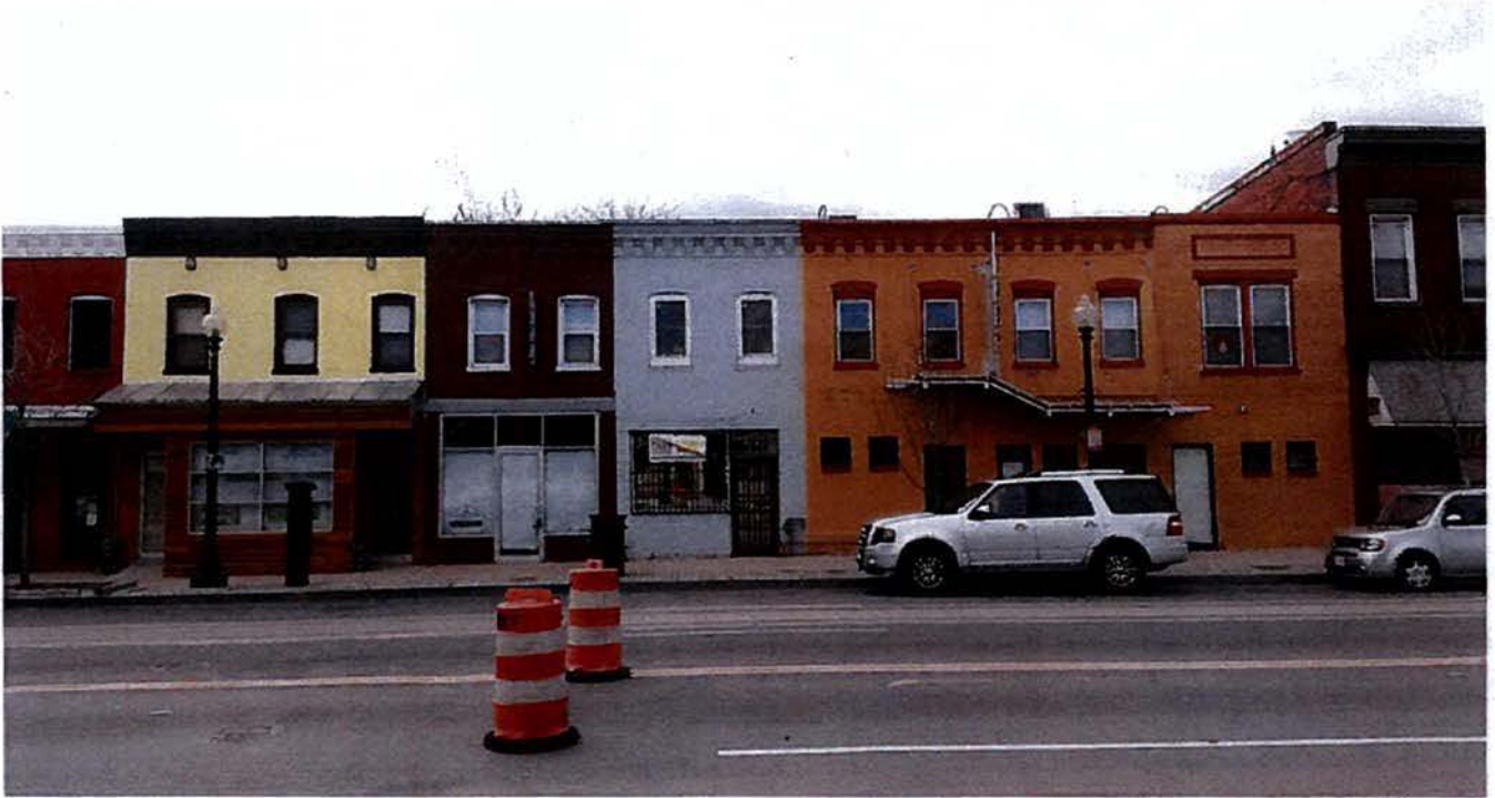
Current view of the Subject Property and neighboring properties, from across H Street
