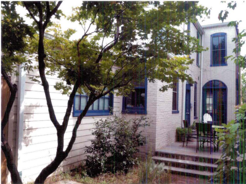
View of 650 C Street NE from rear yard
