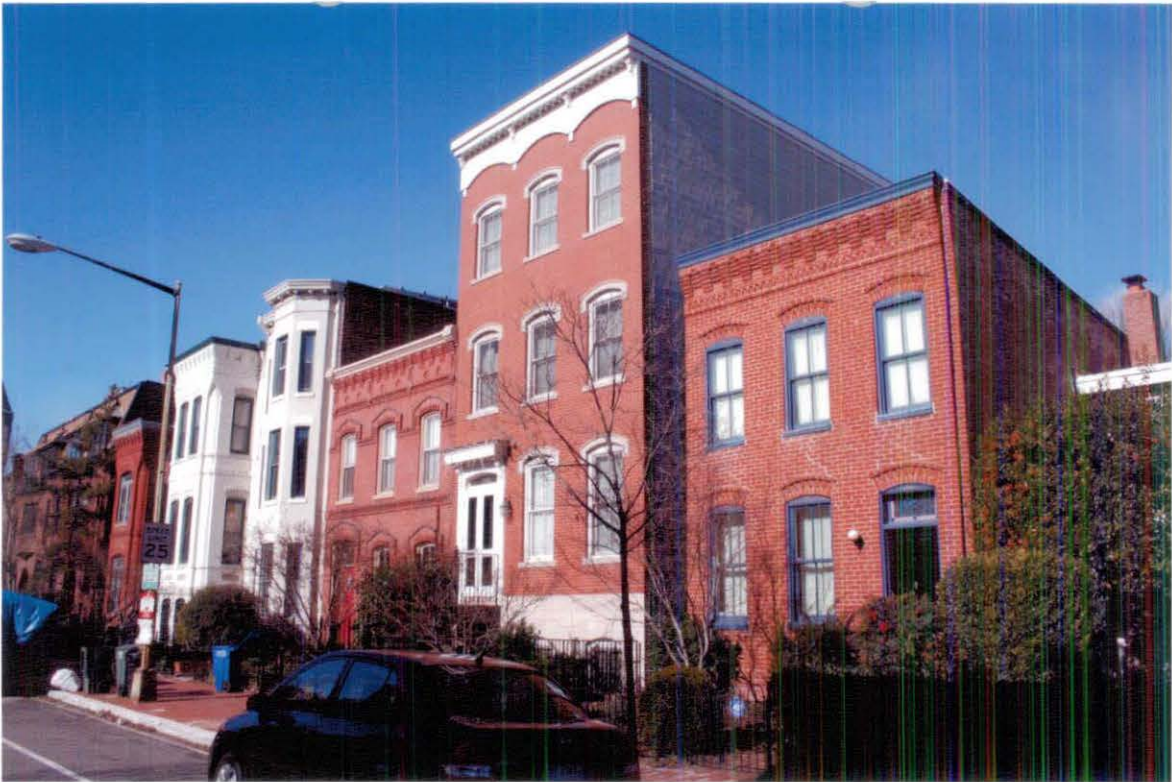
View of 650 C Street NE looking northwest
