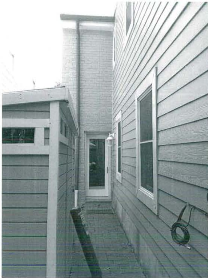
1 EXISTING SIDE YARD AND SHED C-5 SCALE: N.T.S.
