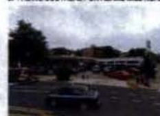
2. FACING EAST ON ADAMS MILL ROAD
