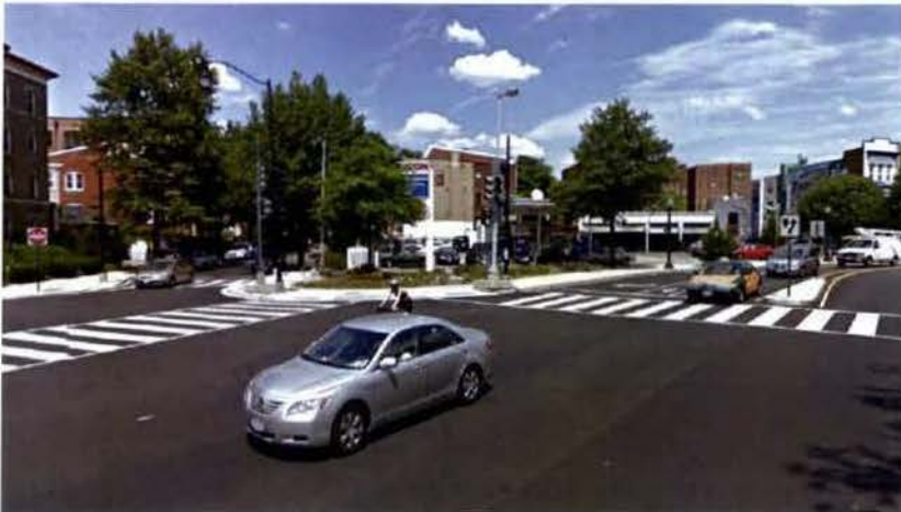
3 CONTEXT PHOTO INTERSECTION OF ADAMS MILL ROAD & LANIER PLACE SCALE: N.T.S.
