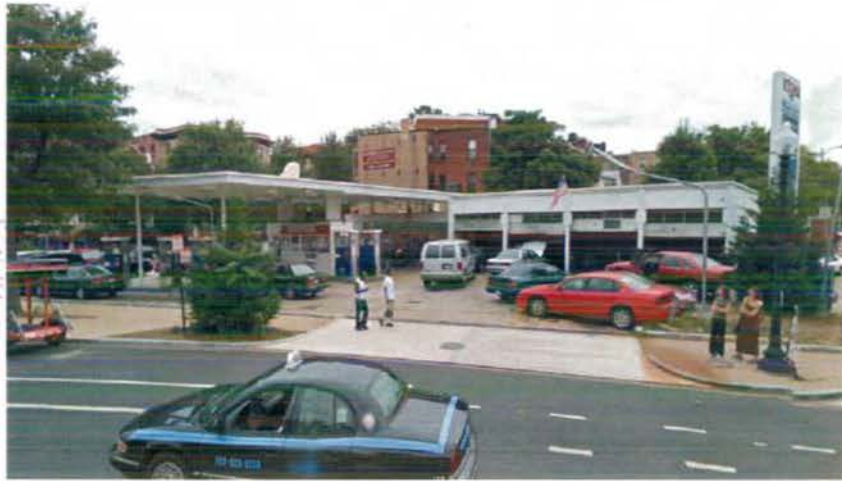
1 CONTEXT PHOTO ADAMS MILL ROAD SCALE: NTS
