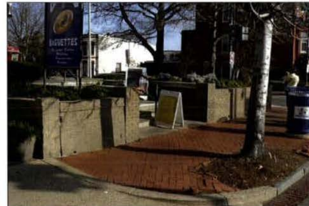
236 Mass Ave retaining wall at sidewalk
