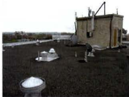
ELEVATOR MACHINE ROOM
