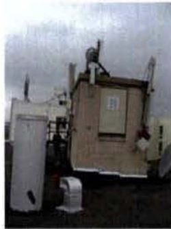
ELEVATOR MACHINE ROOM
