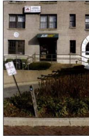
236 Mass Ave west entrance
