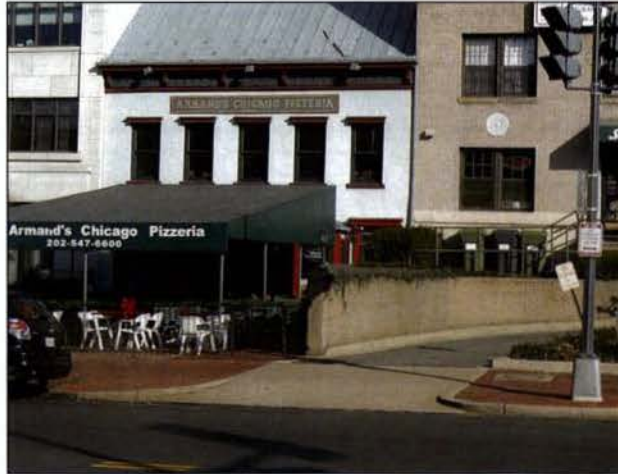
236 Mass Ave driveway
