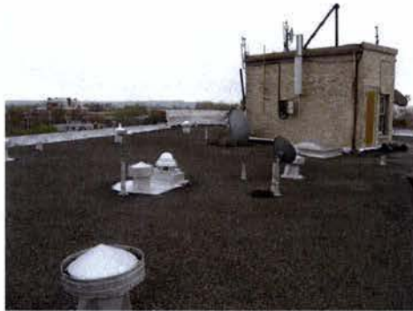
ELEVATOR MACHINE ROOM
