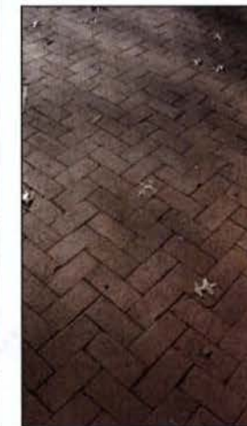
Typical brick paving near site
