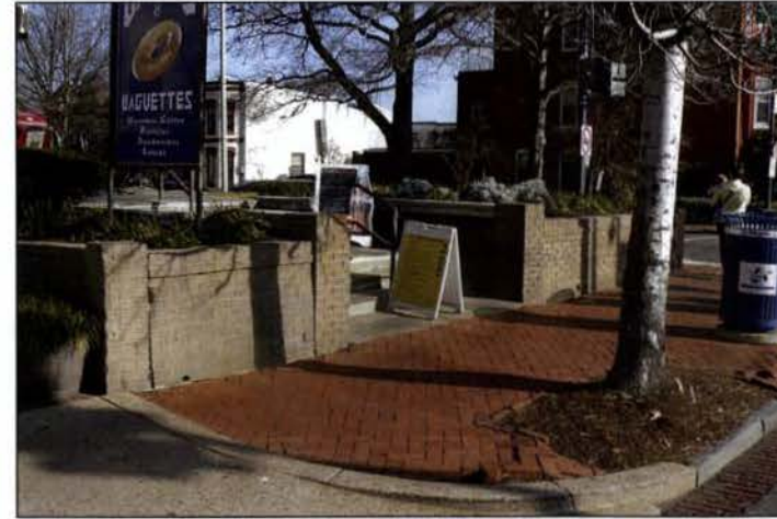
236 Mass Ave retaining wall at sidewalk
