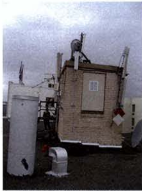
ELEVATOR MACHINE ROOM
