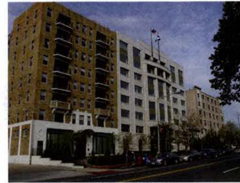
MASS AVE LOOKING EAST
