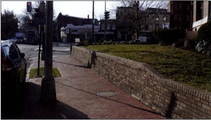
3rd Street sidewalk near corner of Mass Ave
