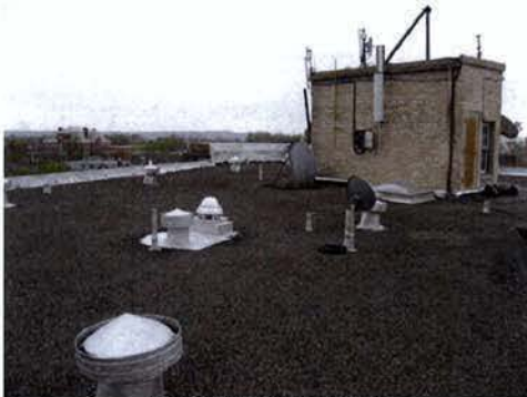
ELEVATOR MACHINE ROOM
