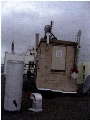
ELEVATOR MACHINE ROOM
