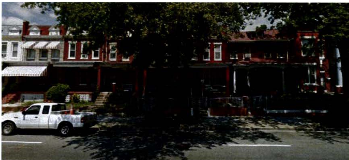
Mansards on the 1200 block of Florida Ave, NE
