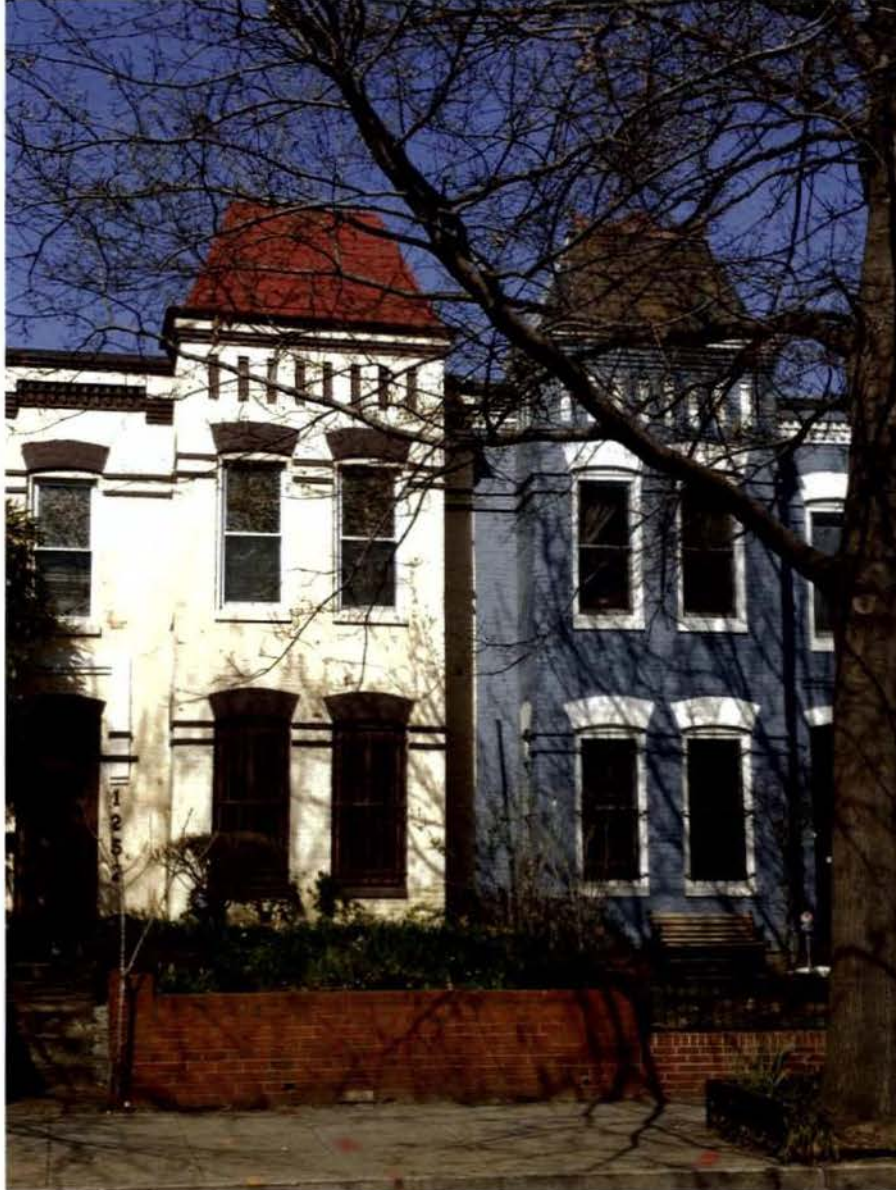
Mansards on the 1200 block of Florida Ave NE
