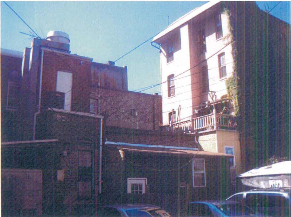
View from the alley of the rear of the Property
