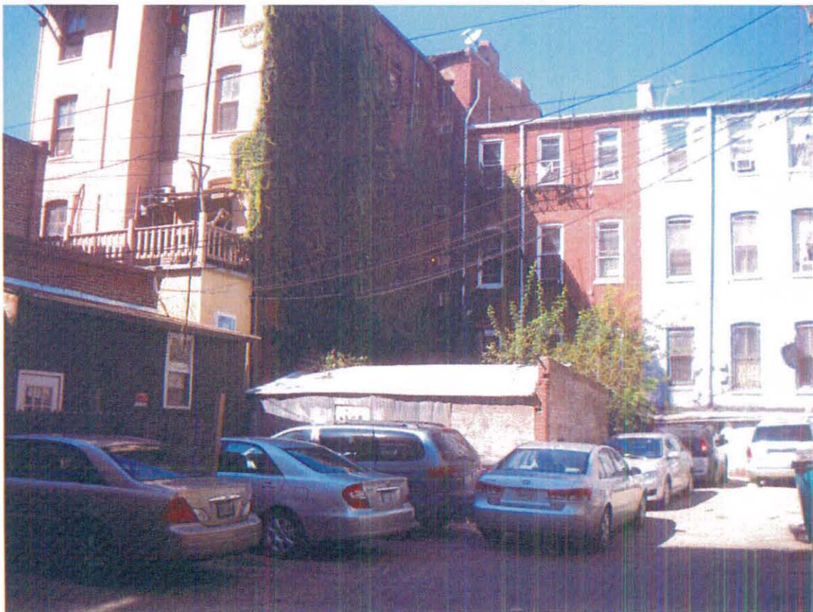
Alley behind the rear of the Property (Property is on the left)
