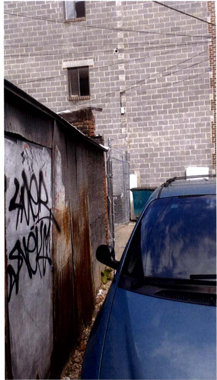
View of the Rear of the Property
