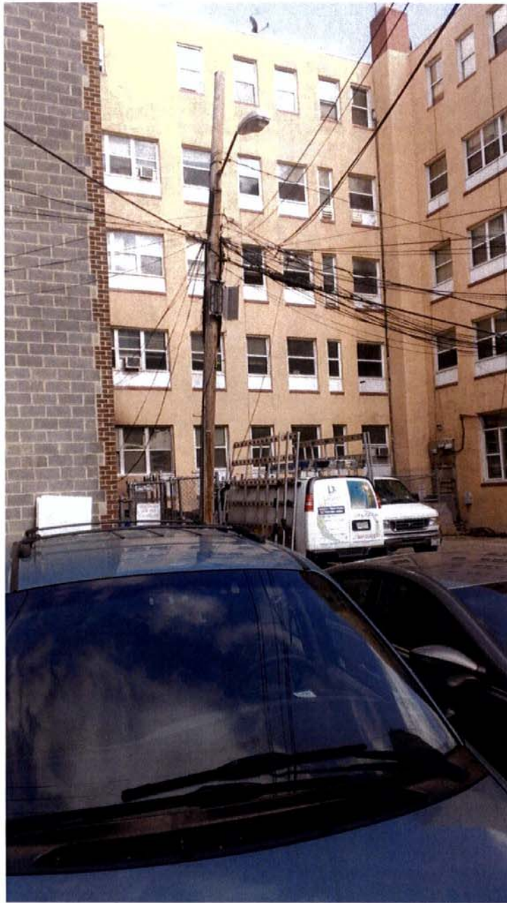
View of the Rear of the Property
