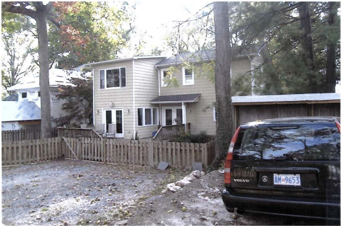
PHOTO #3 AT REAR OF EXISTING HOUSE
