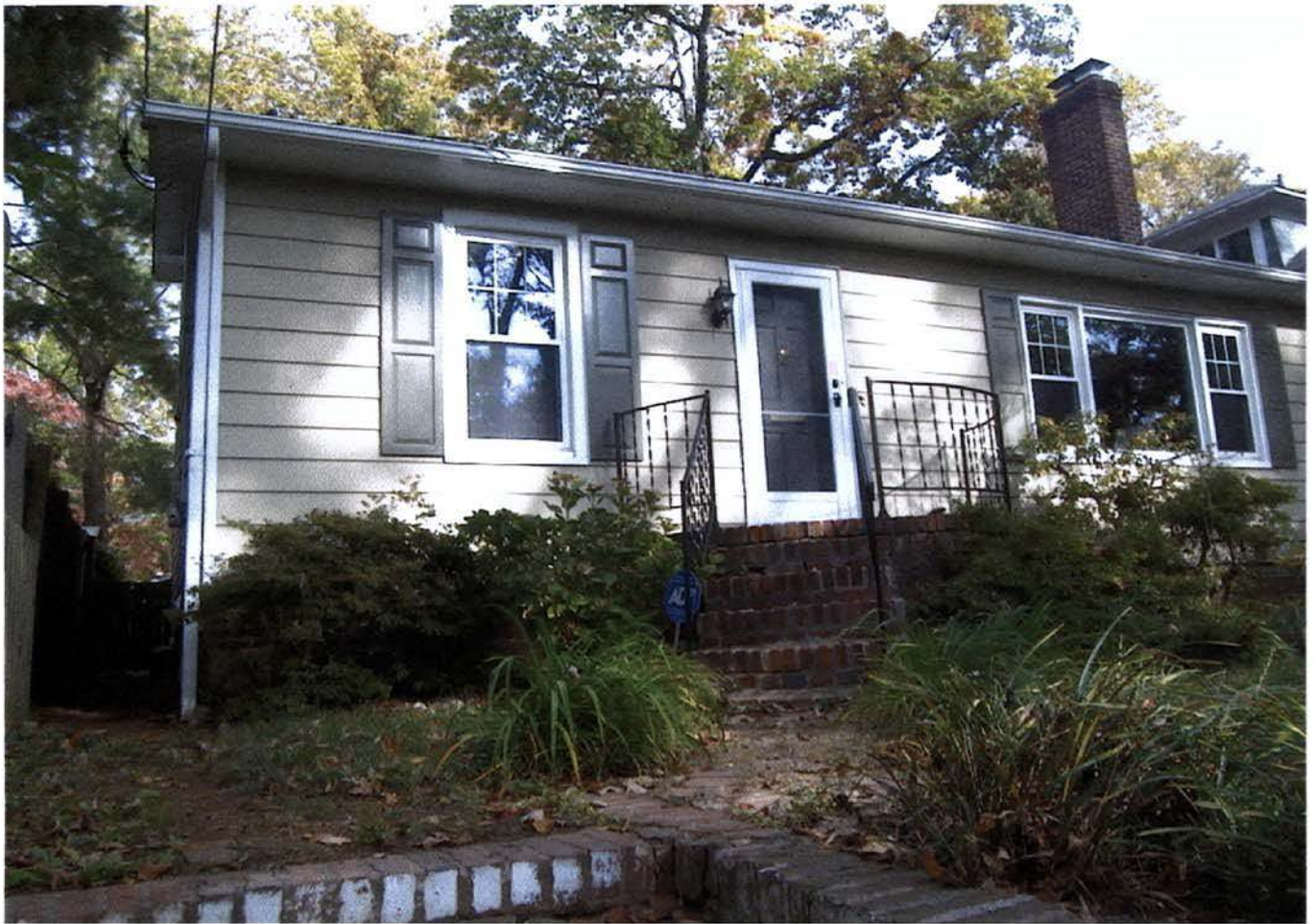
PHOTO #1 AT FRONT OF EXISTING HOUSE
