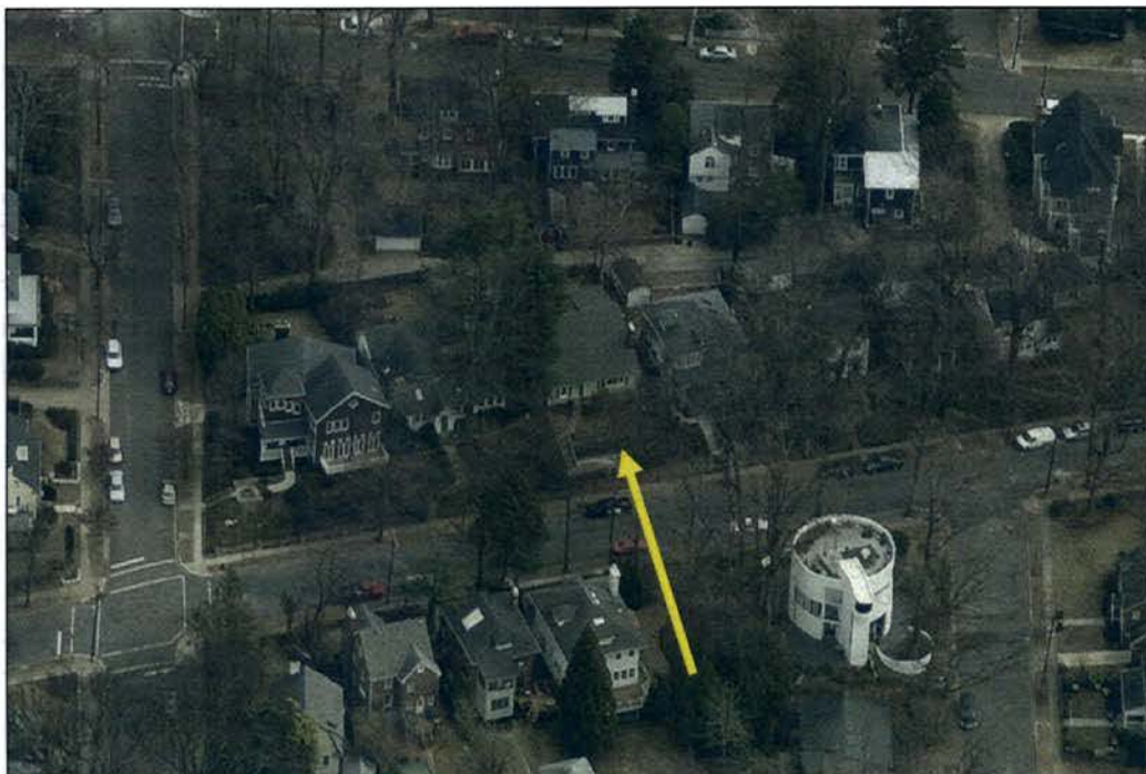
View looking east across Broad Branch Road (subject property identified); Source: OP (2009 image)
