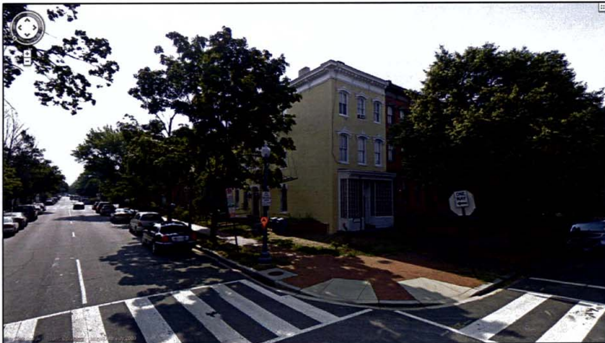
LOOKING SOUTHEAST FROM INTERSECTION OF INDEPENDENCE AVENUE AND 5 TH STREET, SE
