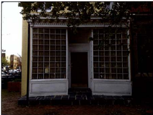
PORTION OF FRONT OF STRUCTURE FACING EAST FROM 5 TH STREET, SE
