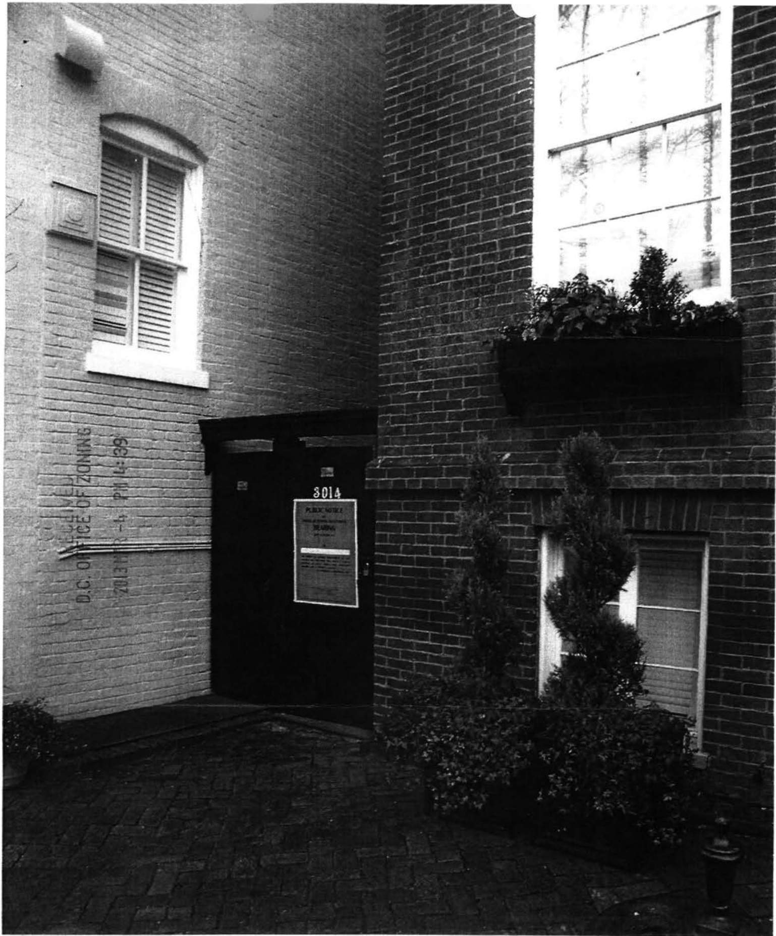
BZA Application #18512 3014 P Street NW Photo #2 From front entry steps looking SE, sign attached to 3014 P Street NW side yard gate
