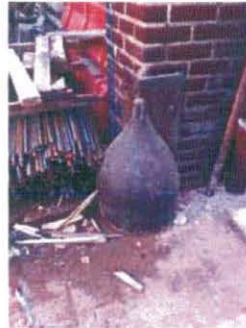
FIGURE 16: CORNER PROTECTION BOLLARD
