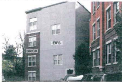
1 CEDAR CROSSING (LOOKING EAST)
