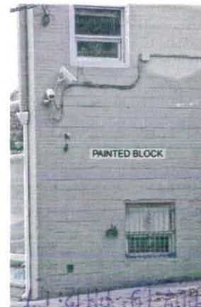
16 LANDIS BUILDING (LOOKING EAST)
