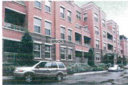
3 GABLES (LOOKING WEST)
