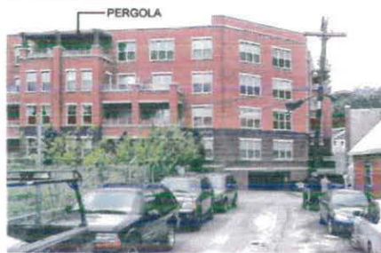
4 ALLEY (LOOKING SOUTH)
