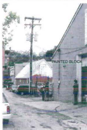
ALLEY (LOOKING SOUTH)
