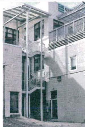
7 LANDIS BUILDING (LOOKING WEST)
