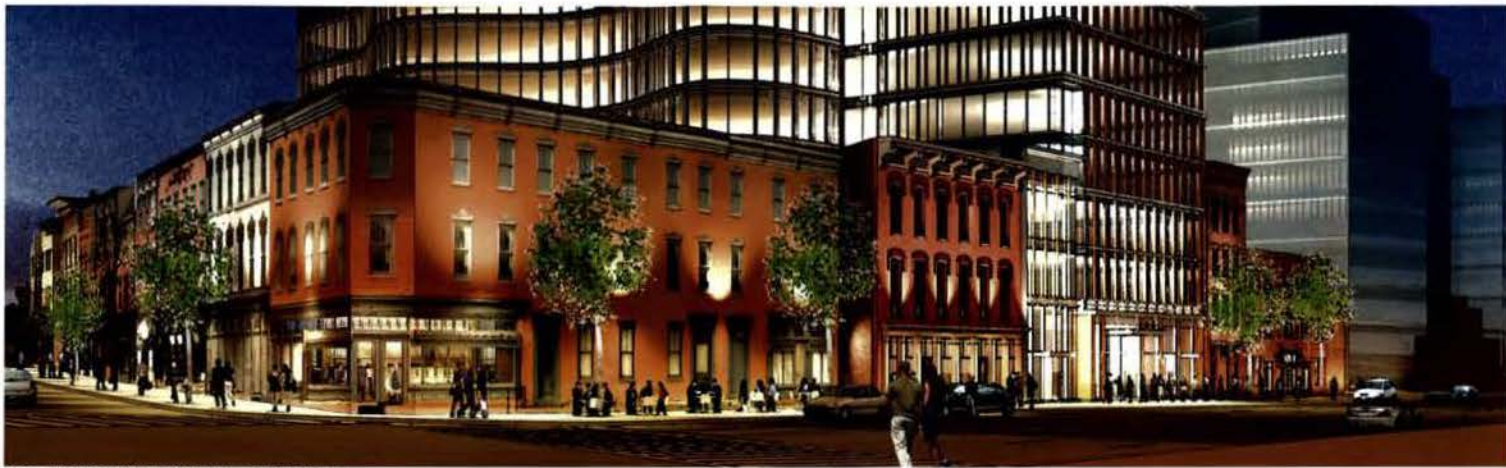
View at Corner of New York Ave. and 7th Street
