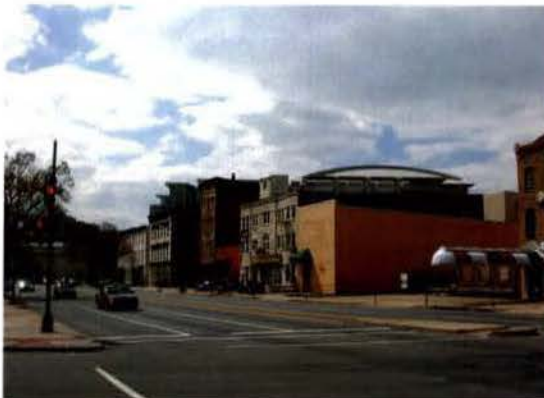
4 View from 6th Street and New York Avenue looking west.
