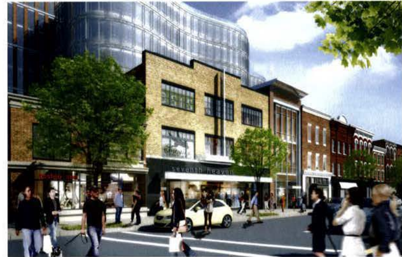
Street View along 7th Street from North
