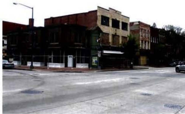
2 View from 7th and L Streets looking southeast.
