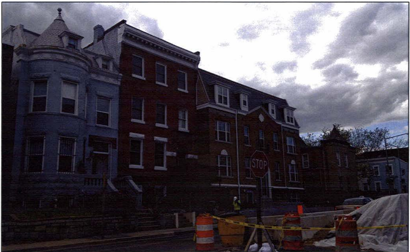
NEIGHBORING FOUR-STORY STRUCTURES
