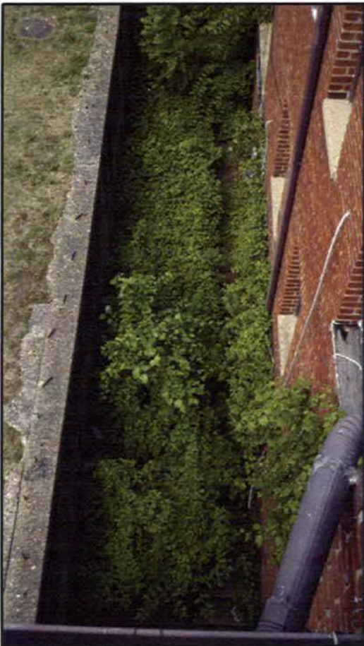
COURT ON SOUTH SIDE OF PROPERTY
