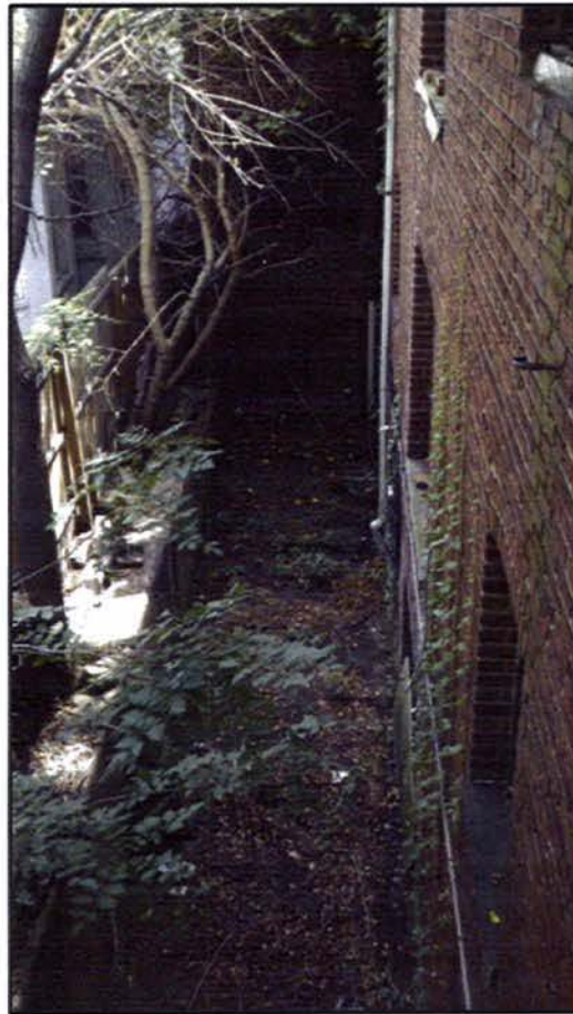
COURT ON NORTH SIDE OF PROPERTY
