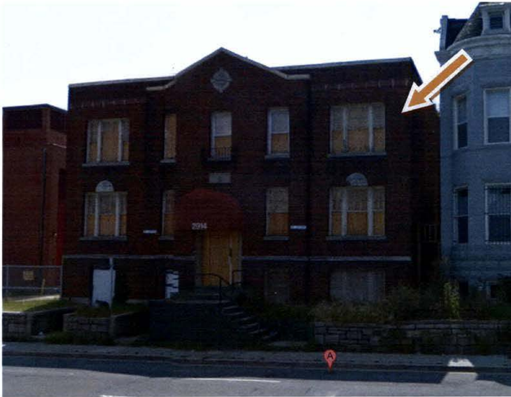
Figure 2: Front of Subject Property
