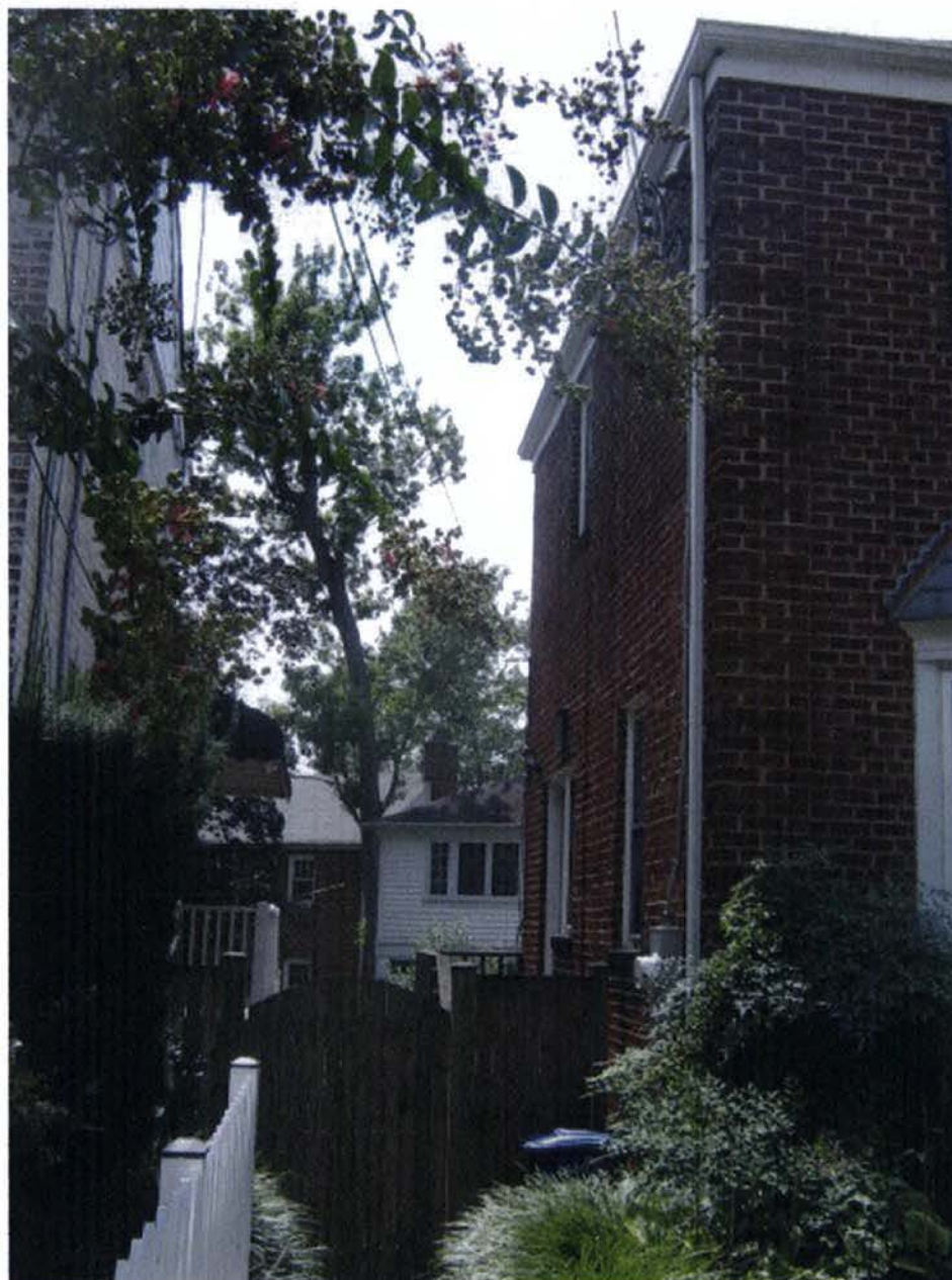
Front/Left View 4764 Reservoir Road, NW For Special Exception/Variance 10-12-12
