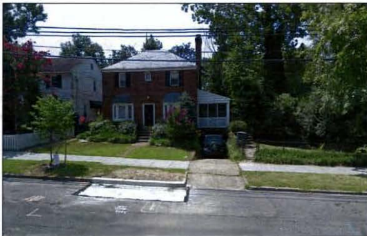
View of the site looking south across Reservoir Road NW. Source: Google Maps 2009.
