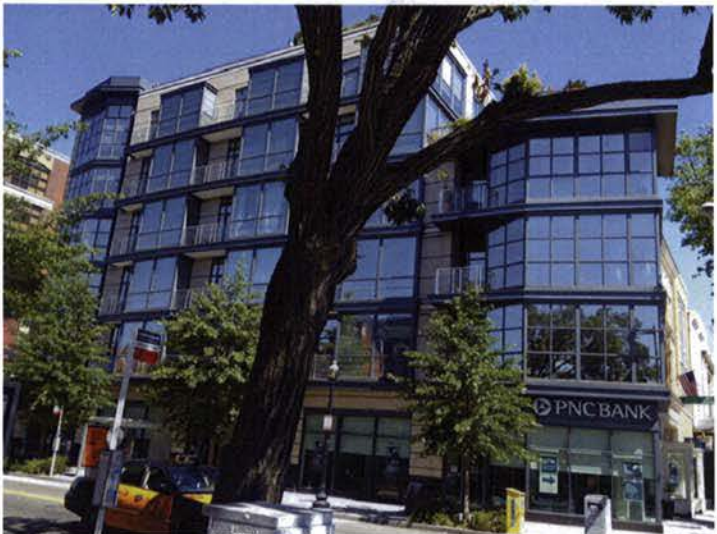
EXISTING NORTHWEST CORNER OF 14TH ST NW AND P ST NW
