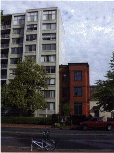
ADJACENT BUILDINGS ALONG RHODE ISLAND AVE
