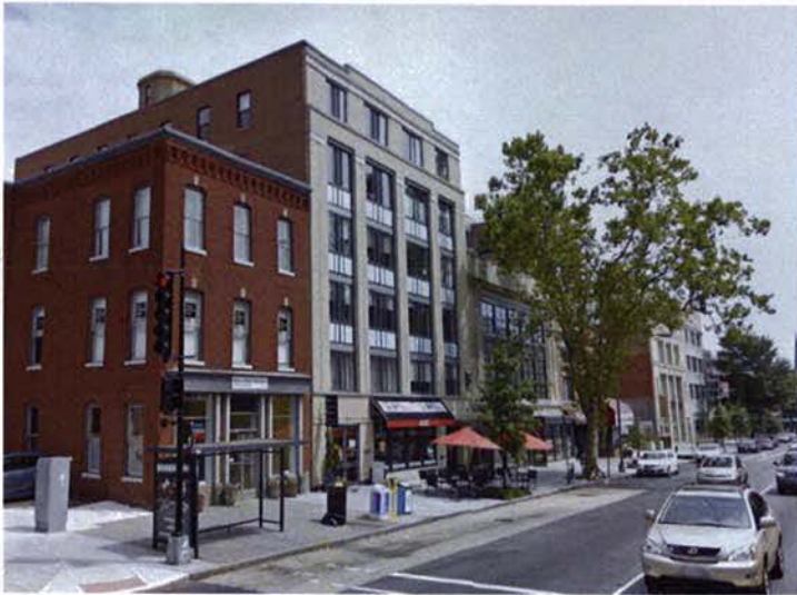
EXISTING SOUTHEAST CORNER OF 14TH ST NW AND Q ST NW
