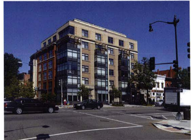
EXISTING NORTHWEST CORNER OF Q ST NW
