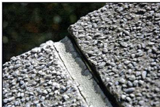
Left: Open sealant joint between two capstones on the North wall of the Tower Top Right: Deteriorated capstone sealant joint on the East wall of the Sanctuary. Bottom Right: Separated capstone sealant joint on the East wall of the Sanctuary.
