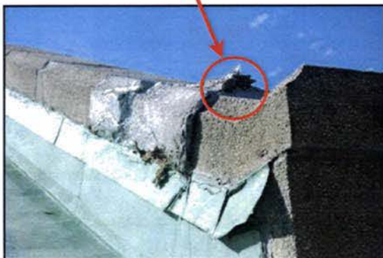
Top Left: Coated capstone has been completely destroyed. Bottom Left: View of coated capstone from NW corner of the Sanctuary. Right: Severely deteriorated capstone on the SE corner of the Sanctuary.
