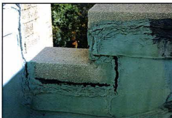
Left: Open sealant joint between two capstones on the North wall of the Tower Top Right: Deteriorated capstone sealant joint on the East wall of the Sanctuary. Bottom Right: Separated capstone sealant joint on the East wall of the Sanctuary.
