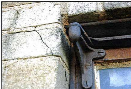
Top Left: Rusted steel casement window and cracked, deteriorated and missing glazing. Bottom Left: Rusted steel header above casement window has started to expand and crack surrounding brick. Right: View of heavily deteriorated glazing on rusted steel casement window.
