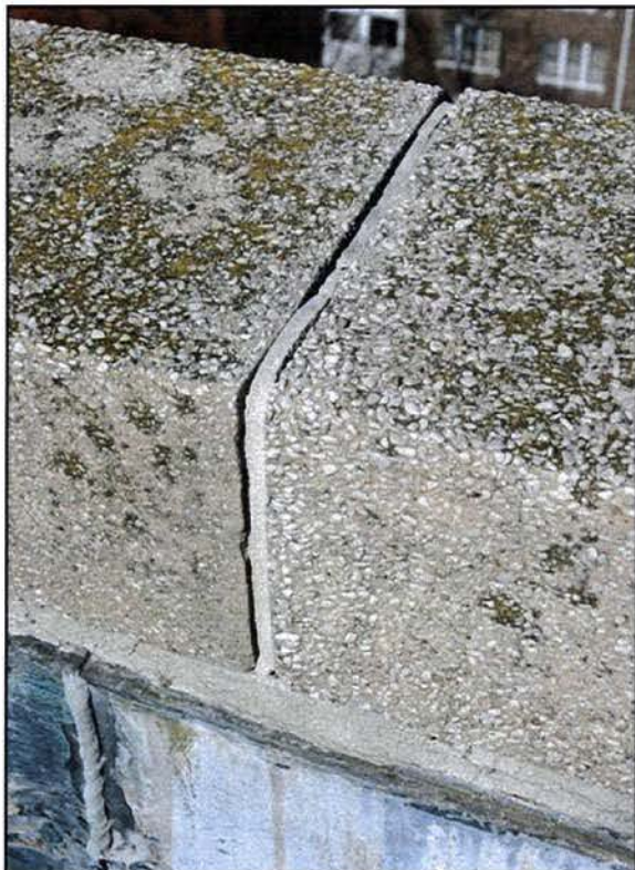
Left: Open sealant joint between two capstones on the North wall of the Tower Top Right: Deteriorated capstone sealant joint on the East wall of the Sanctuary. Bottom Right: Separated capstone sealant joint on the East wall of the Sanctuary.
