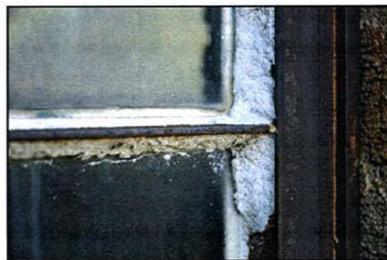
Top Left: Rusted steel casement window and cracked, deteriorated and missing glazing. Bottom Left: Rusted steel header above casement window has started to expand and crack surrounding brick. Right: View of heavily deteriorated glazing on rusted steel casement window.
