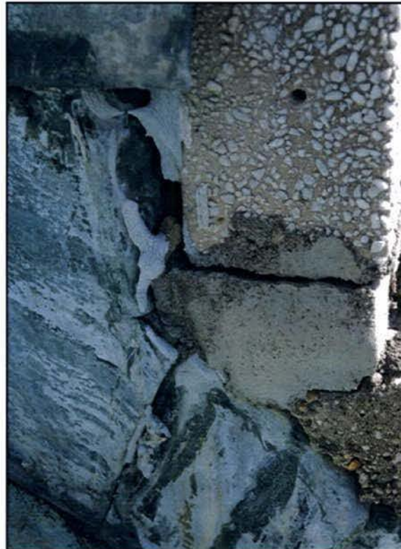
Bottom Left: Improperly sealed and installed flashing on the back side of the capstones on the West sanctuary wall.
