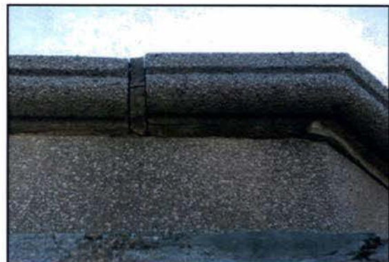
Bottom Right: Many stone mortar joints on the tower are completely deteriorated. Large chunks of mortar have simply fallen out the joints.
