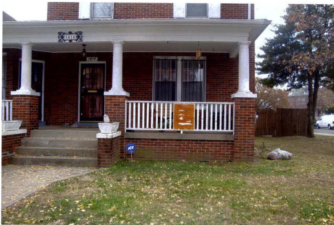
Photograph 2 - street frontage to 15th Street, NW
