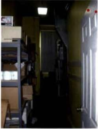
Interior masonry walls
